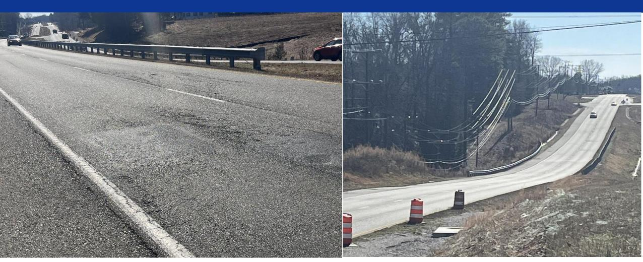
Segregation deeper in the pavement structure – BM Placement on 164 in Hampton Roads
