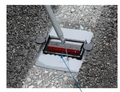
Fill the plunge cut until the PIM holder's "teeth" are fully covered
