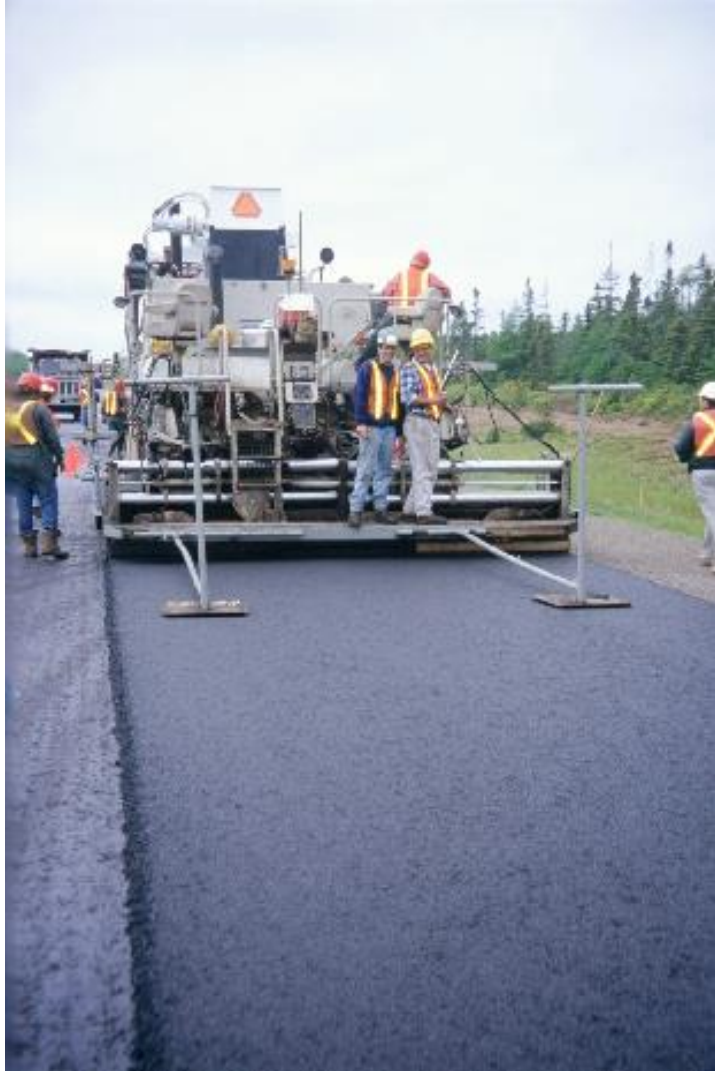
CONSTRUCTION OF DURABLE LONGITUDINAL JOINTS
